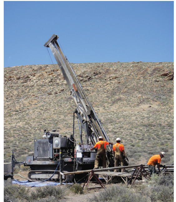
Drill Rig at the North Bullfrog project
